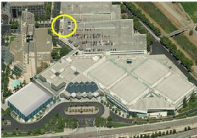
1 st Floor of the Parking Garage near entrance on Bunker Hill
